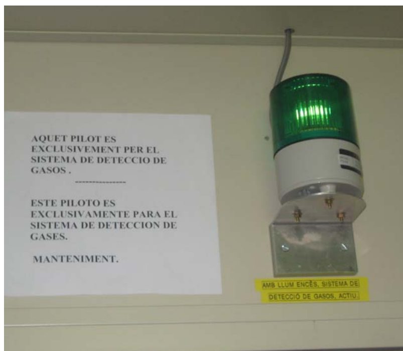
Fig. 04. Gas detection indicator in the pre-SAS.
